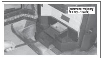
Figure 47 - Lower Ash Pan, Profile 30 INS-2
